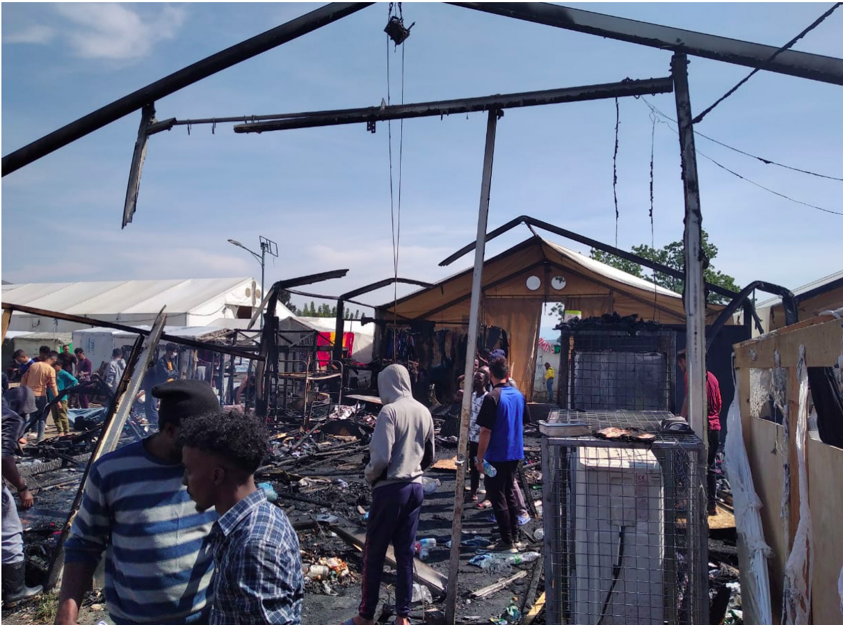
Fig. 9 & 10 Residents walking through destroyed Structures after the Fire on April 18, 2020
