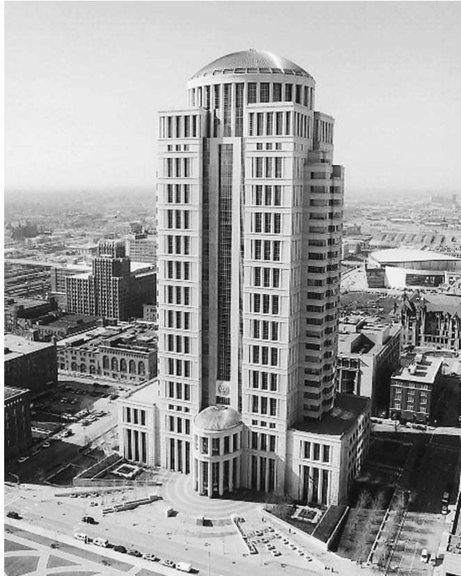
Thomas F. Eagleton Federal Courthouse, St. Louis, Missouri, 2000. Architects: Hellmuth, Obata + Kassabaum, Inc. Figure 39.
