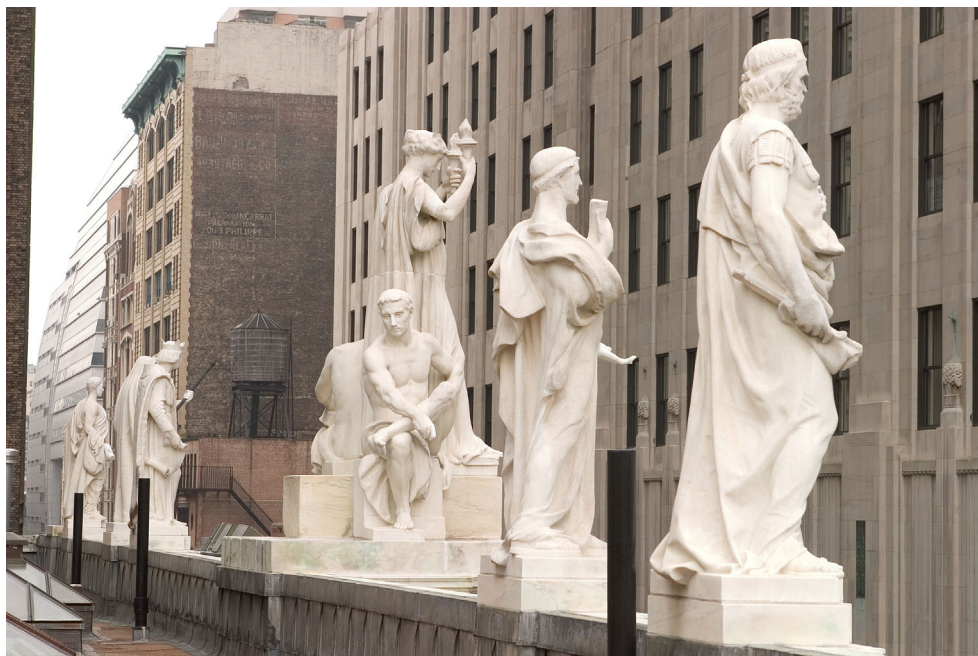
Statuary on the roof of the New York State Supreme Court, Appellate Division, First Judicial Department, New York City, 1900. Figure 28.
