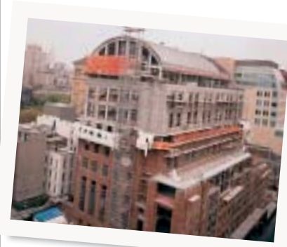
The new building takes shape. The view on December 2, 2002, (left) and the progress five months later on May 6, 2003 (bottom). [Credit: Bernstein Associates (Harrison, NY) for Plaza Construction] Top: The final piece of structural steel adorned with the U.S. and NYU flags is lifted to the roof of the new building at the Topping Out Ceremony on December 6, 2002.
